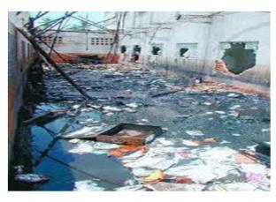
This photo shows the top floor of the building. After consuming the fire the class room partition and the roof. Here there is no door, window, proper ventilation or escape route for each class room.
