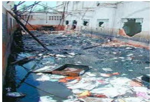
*This photo shows the top floor of the building. After consuming the fire the class room partition and the roof. Here there is no door, window, proper ventilation or escape route for each class room.*
