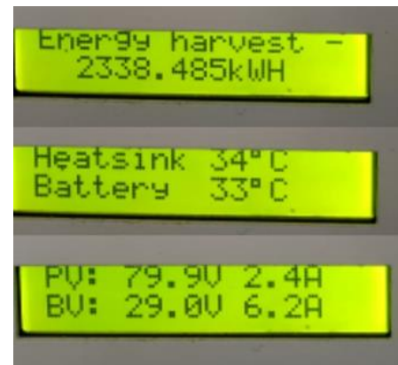
Fig.14 Display of panel voltage, current, Battery voltage, current, battery temperature
