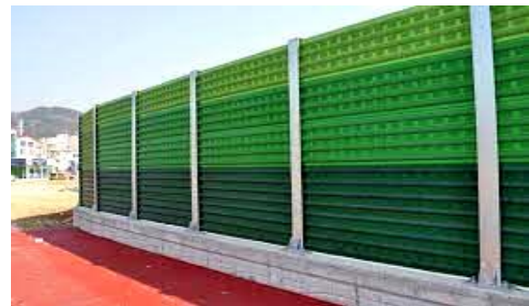
b) Steel Material Interference Type Sound Barrier Fig. 2 Steel Material Interference Type Sound Barrier
