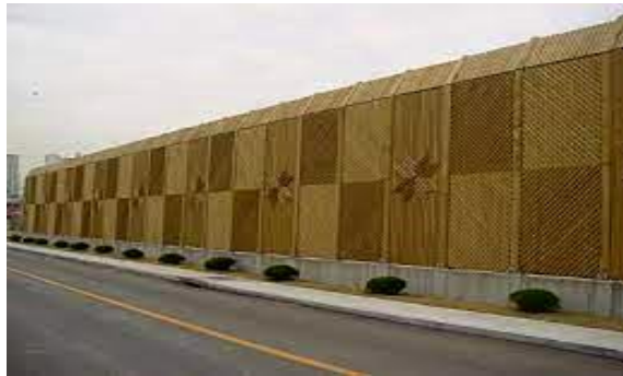
b) Wood Material Interference Type Sound Barrier Fig. 3 Wood Material Interference Type Sound Barrier
