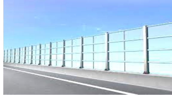
b) Flat Type Transparent Sound Barrier Fig. 1 Flat Type Transparent Sound Barrier
