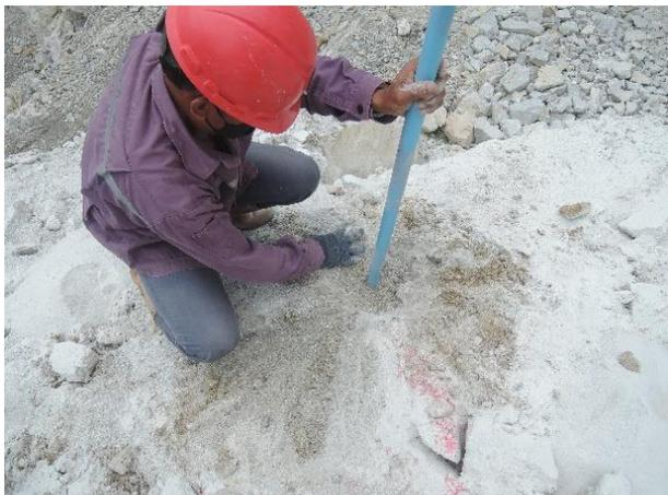
**Fig. 8 Natural rubber latex blasting process**
