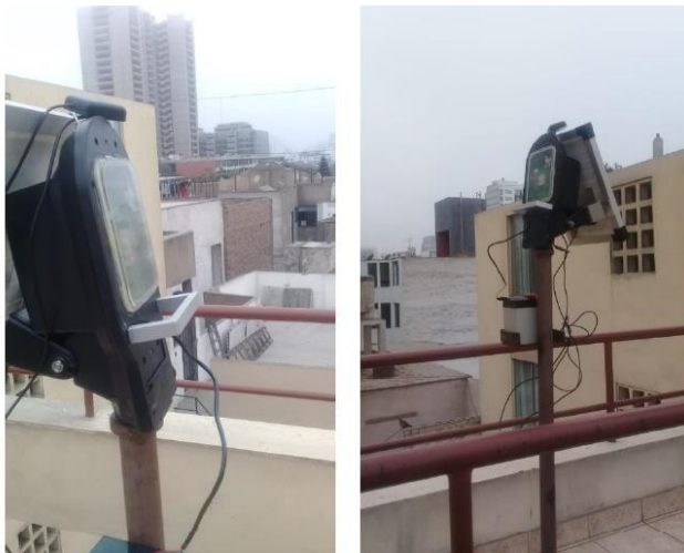
Fig. 22 Location on Building Roof
