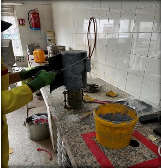
Fig. 3 Impregnation of the CFRP using the resin on the concrete support
