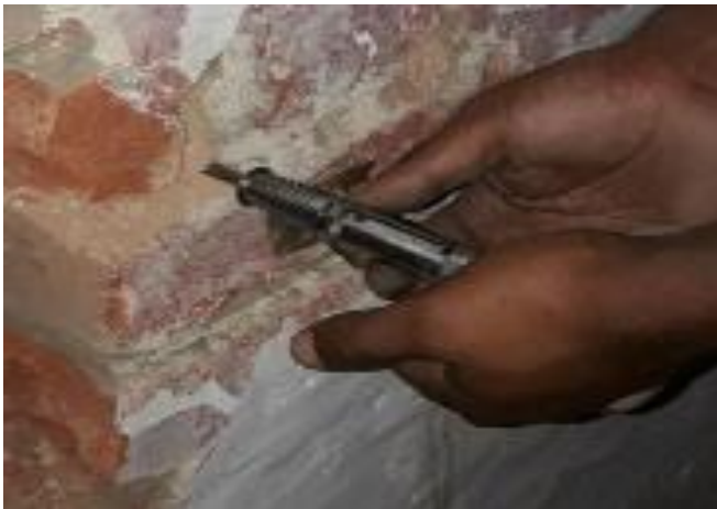
Fig. 10 Pocket penetrometer test
