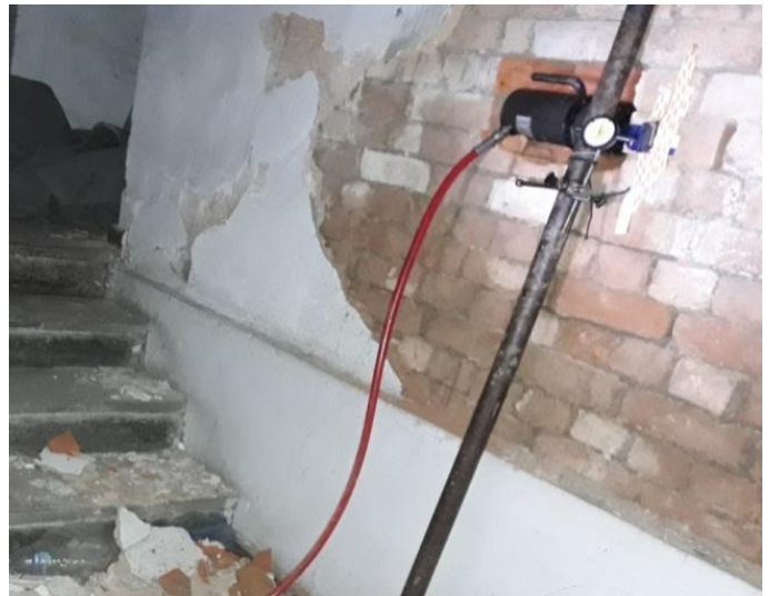
Fig. 8 In-situ shear test
