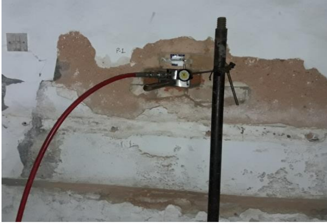
Fig. 9 In-situ Compression test
