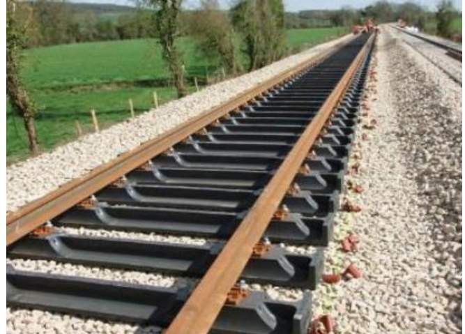
Fig. 7 Recycle plastic sleeper [17]
