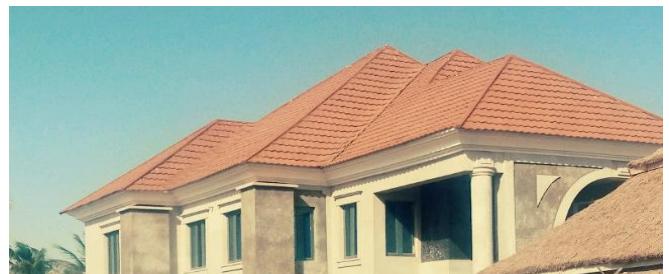
Fig. 13 Multi-level roof in a residential building in Ungwan Dosa, Kaduna
