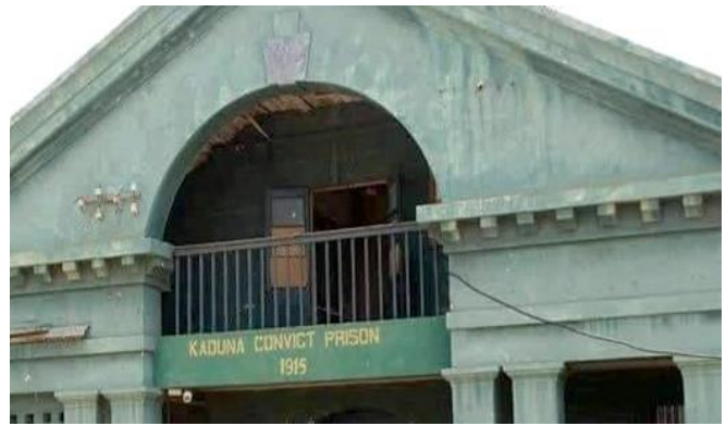
Fig. 10 Pediment and entablatures on the front façade of Kaduna Prison Source: Alabi (2020)
