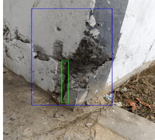
Fig. 14 Detection of Exposed Steel and Spalling
