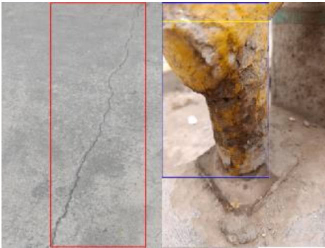
Fig. 13 Crack and Corrosion Detection
