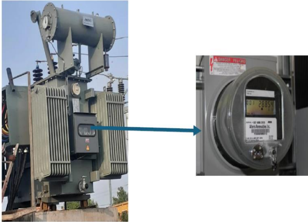
Fig. 3 Energy meter built in the transformer to monitor total energy consumed by the consumers
