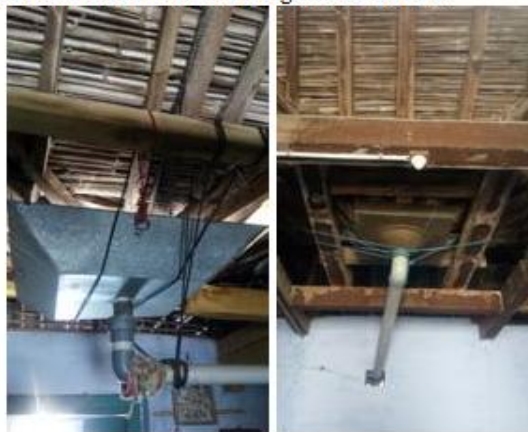
Figure 14. Manduwa transformed from open cut-out to piped concealed trough
