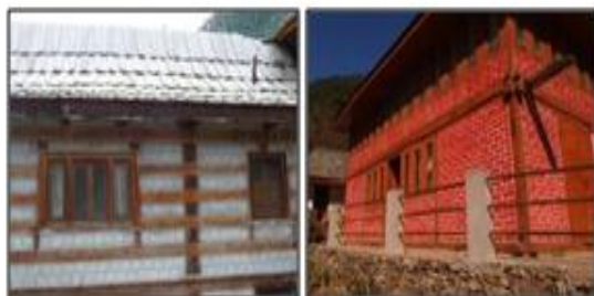
Figure 7. Absence of Kath Kuni style with use of concrete blocks
