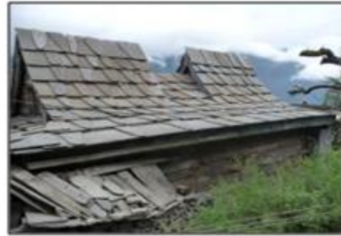
Figure 6. Steep Pitched roof
