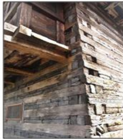
Figure 2. Kath Kuni construction
