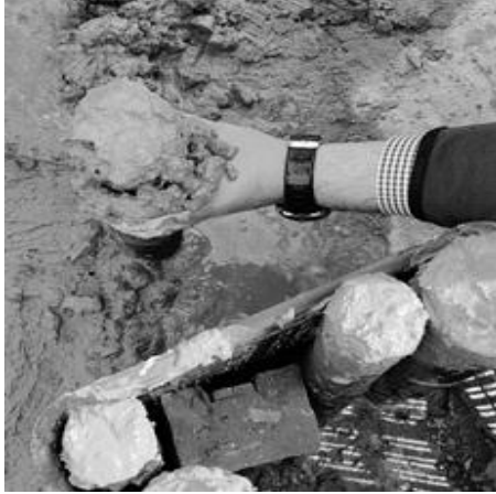
Figure 2. Filling of concrete
