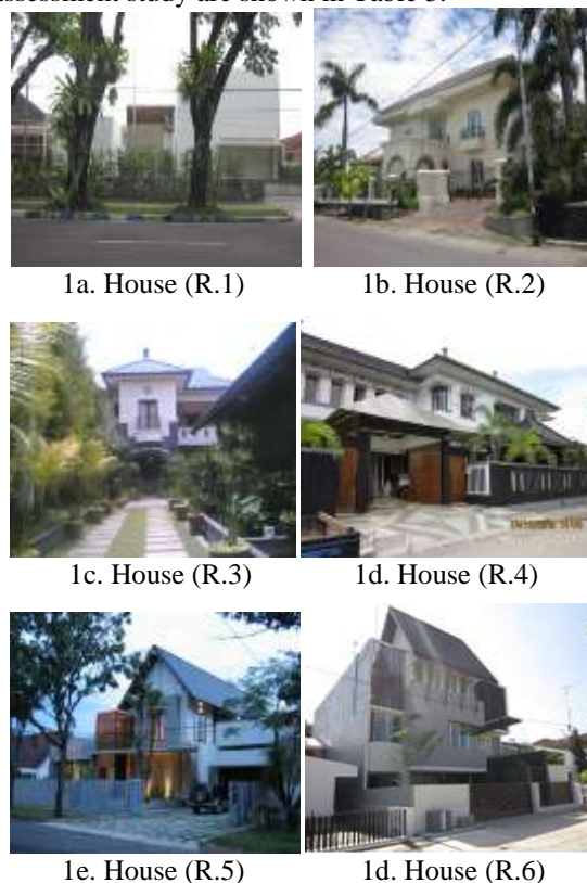
Fig 1. Photo of the front view of the building assessment residence
