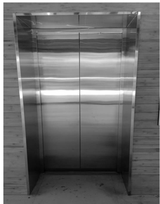
Fig. 3: Installation lift door and ceiling.
