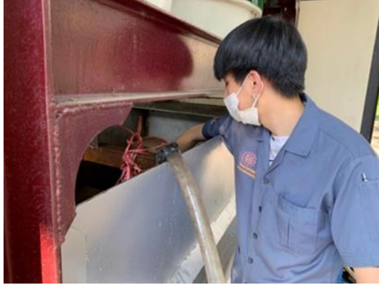
Fig. 2 Pumping out old water from the cooling tower
