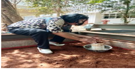
Fig 5: Taking soil in the foundation tub that has been compacted for testing physical characteristics and compaction testing
