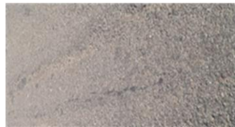
Fig. 6. Slippage cracking
