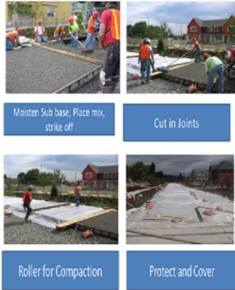
Figure 2: Placement of Pervious Concrete for Roadway
