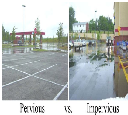
Figure 3: Pervious Vs Impervious Surface
