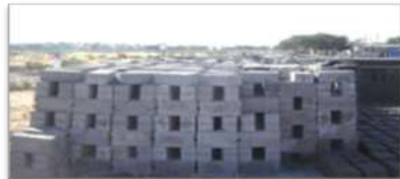
Figure 7: Blocks stacked at plant
