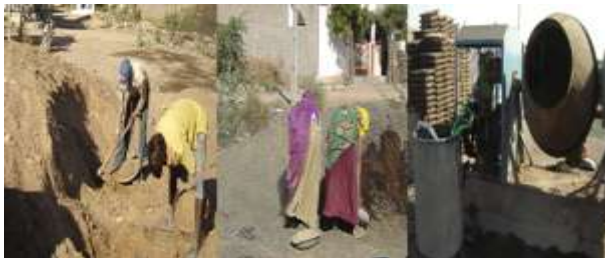
Figure 4: Volume batching of materials and tilted concrete mixture
