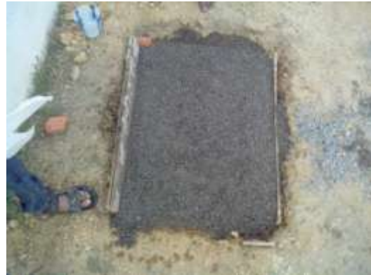
Fig.5. After placement and finishing
