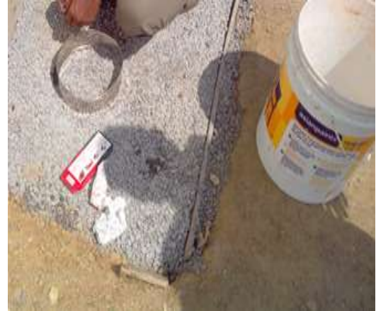
Fig.8. Infiltration ring is placed
