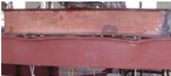
Figure 14 Buckling under the loading point
