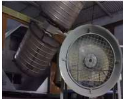
Fig.6 Forced Cooling of hot moulds by fans
