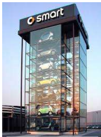
Fig. 5 Tower Type System
