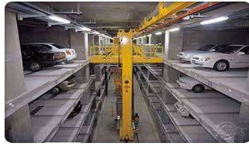
Fig. 8 Crane Parking System
