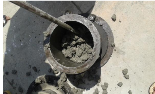
Fig 2: Casting of specimens
