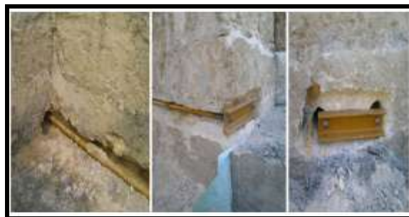
Fig. (17): Tendons installed to masonry wall.
