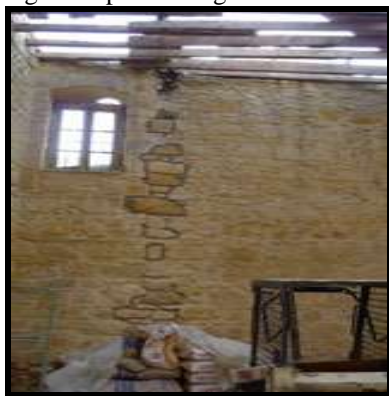
Fig. (12): Crack restoration with tie-stones.
