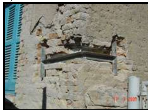
Fig. (14): Reinforcing of the corner by galvanized metal element.
