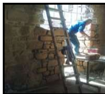
Fig. (10): Reconstruction using tie-stones.
