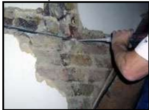
Fig. (13): Crack widening by removing the mortar, loose stones and gallets.
