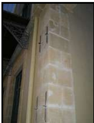
Fig. (15): Typical steel connectors for stone masonry.
