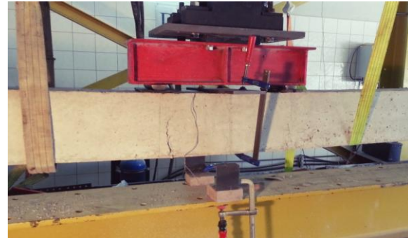
Fig 8: Crack in prestressed plain concrete.
