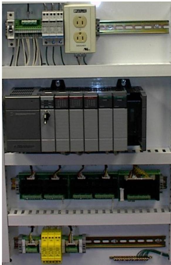
Fig: Control panel with PLC (grey elements in the center). The unit consists of separate elements, from left to right; power supply, controller, relay units for in- and output.
